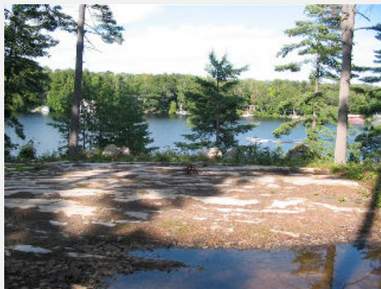
Cleared Building Site
