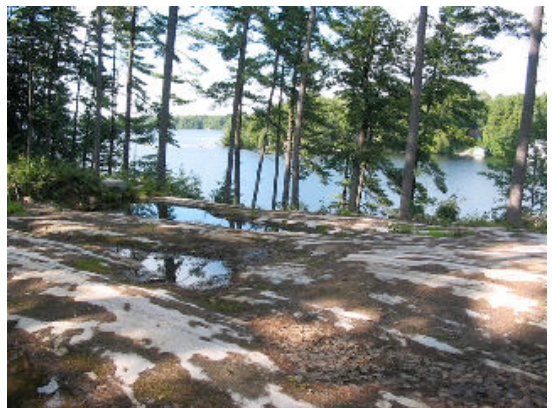
Cleared Building Site
